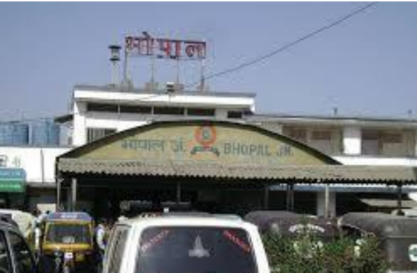
From Bhopal Junction Railway Station
